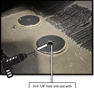
Drill 7/8" hole and seal with RTV Silicone
