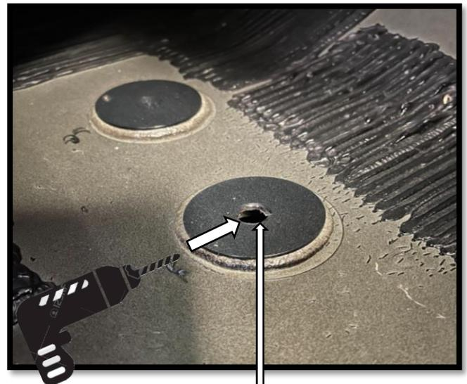
Drill 7/8" hole and seal with RTV Silicone
